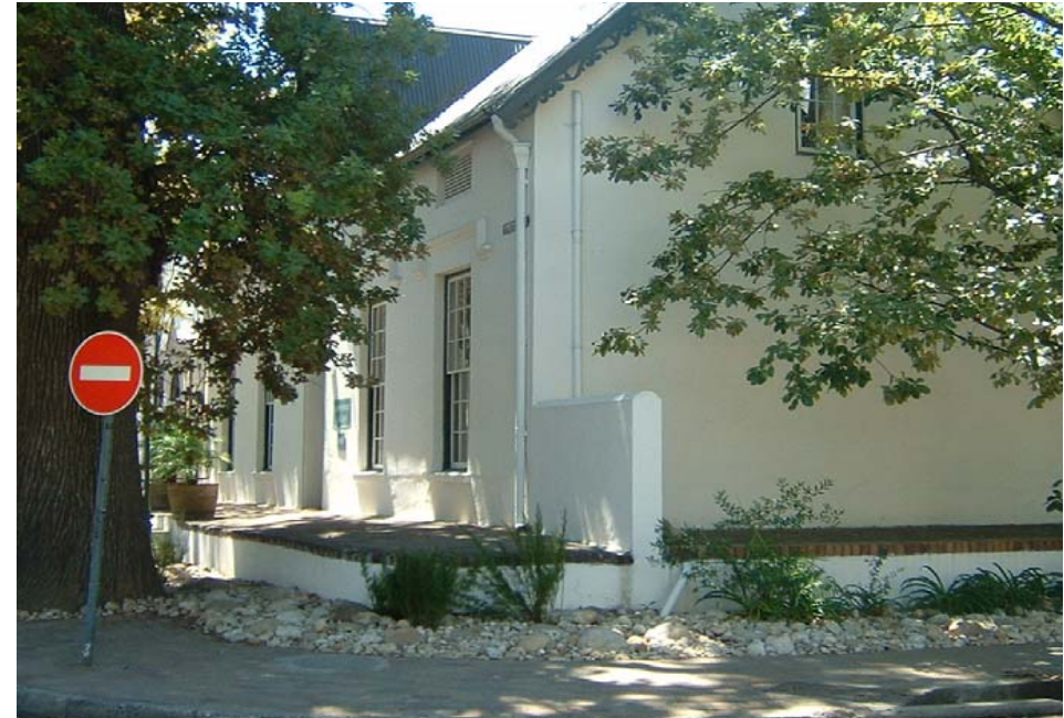
Figure 8.14 Appropriate architectural character
